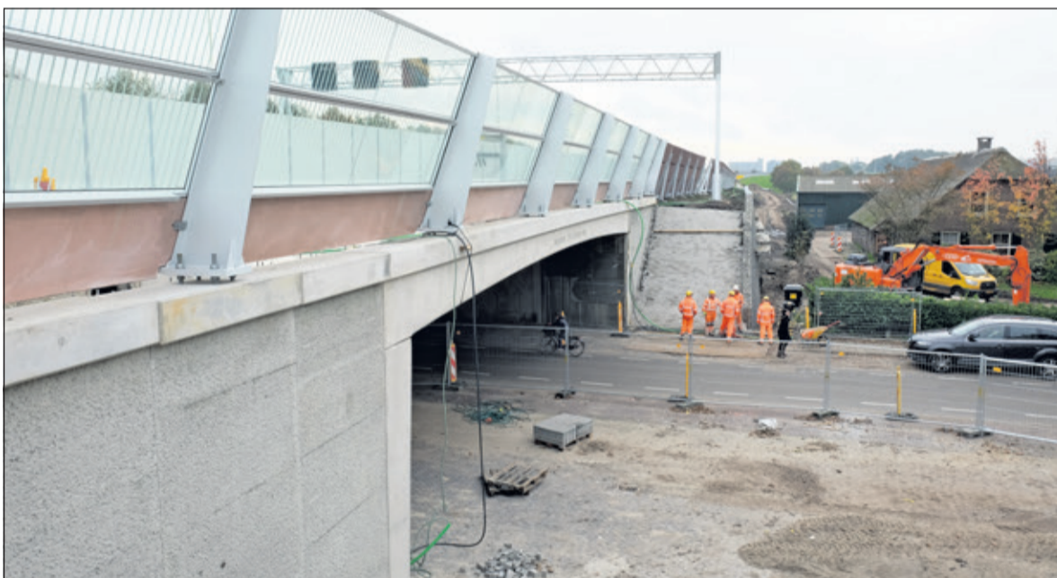
Viaduct Groenekan nadert voltooiing.
